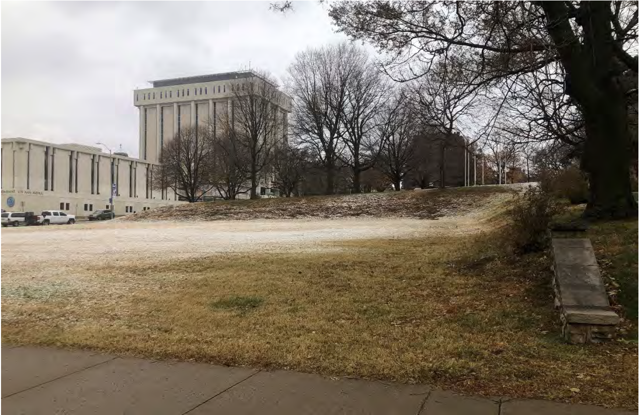
Figure 6. Site Photograph of 810 North 6th Street looking southwest from North 6 th Street (provided by Planning Staff).
