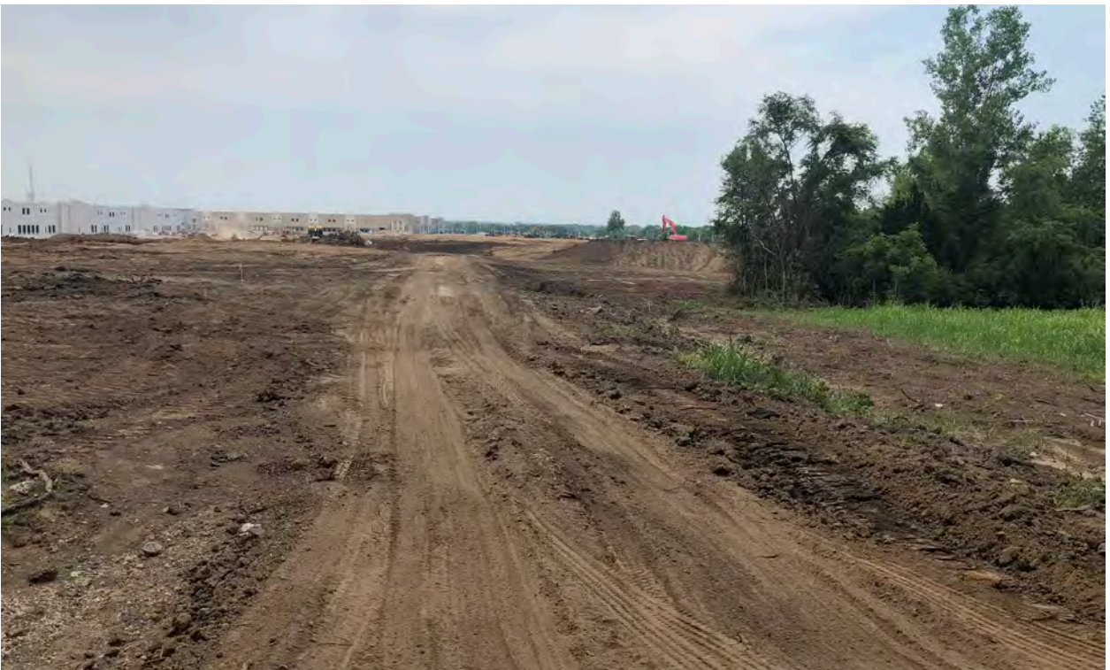
Figure 2. Site photograph of Turner Logistics Center (provided by Planning Staff).
