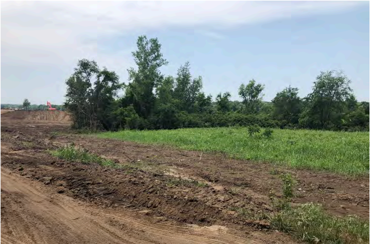
Figure 1. Site photograph of Turner Logistics Center (provided by Planning Staff).
