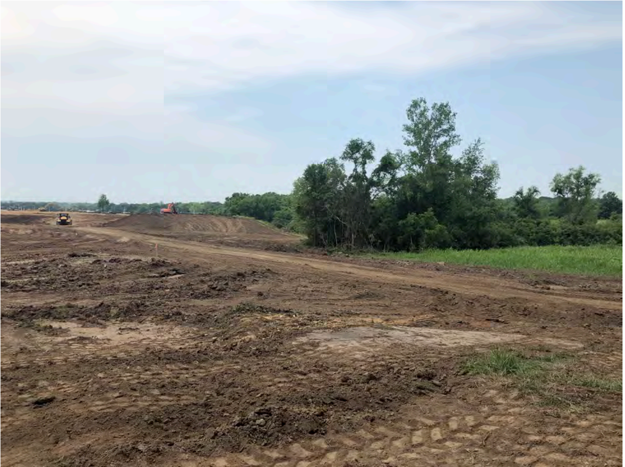
Figure 3. Site photograph of Turner Logistics Center (provided by Planning Staff).
