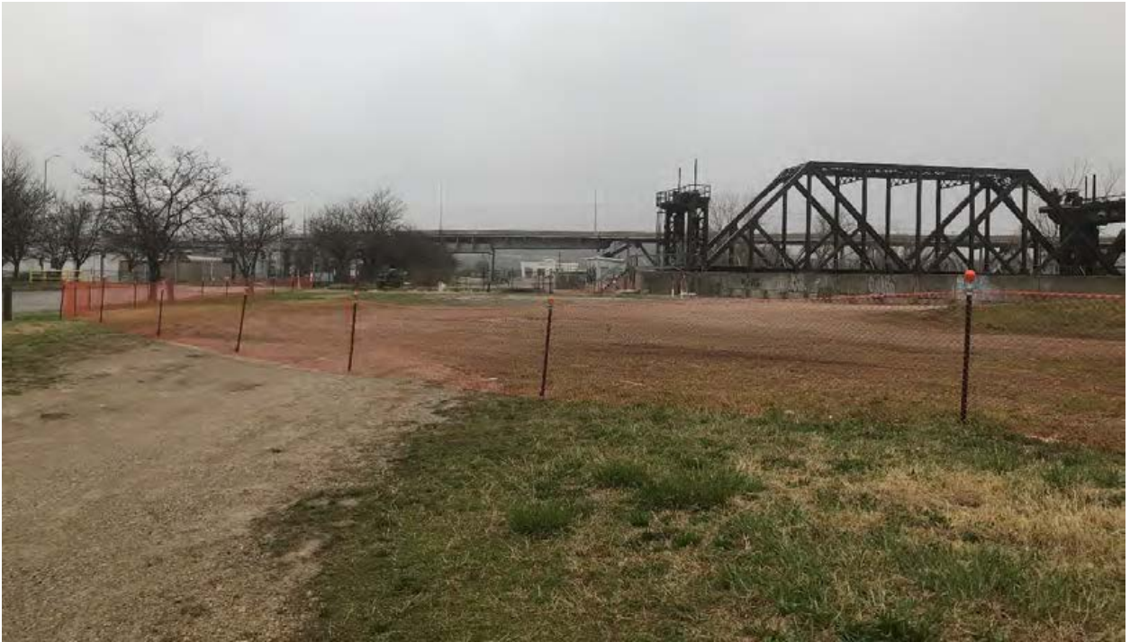
Figure 3. Site Photograph of the Rock Island Bridge looking southwest from 200 South James Street (provided by Planning Staff).
