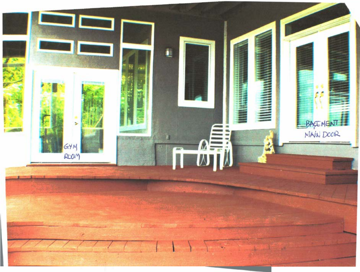
BASEMENT MAIN DOOR & GYM ROOM/STORAGE
